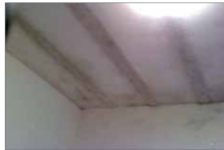
These images clearly show that the cold spots caused by thermal bridges exactly coincide with mold development.
